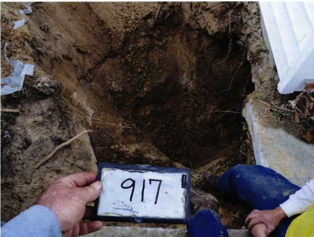
Picture 2: UST 917Barracuda excavation.
